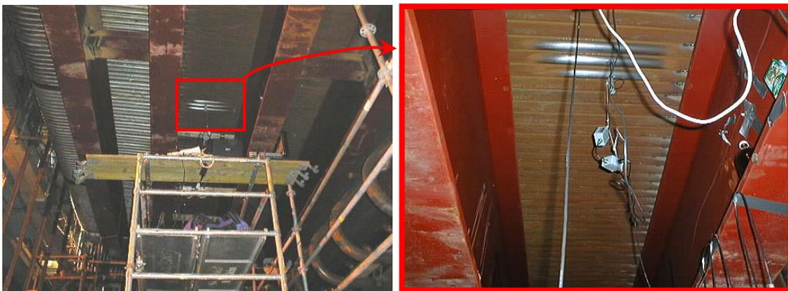
Figure 9. Measurements were performed at the bottom wall of the recovery boiler (left). Zoomed view at right.
