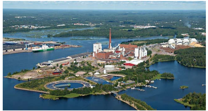
Sunila Mill in Kotka. Photo: Stora Enso
