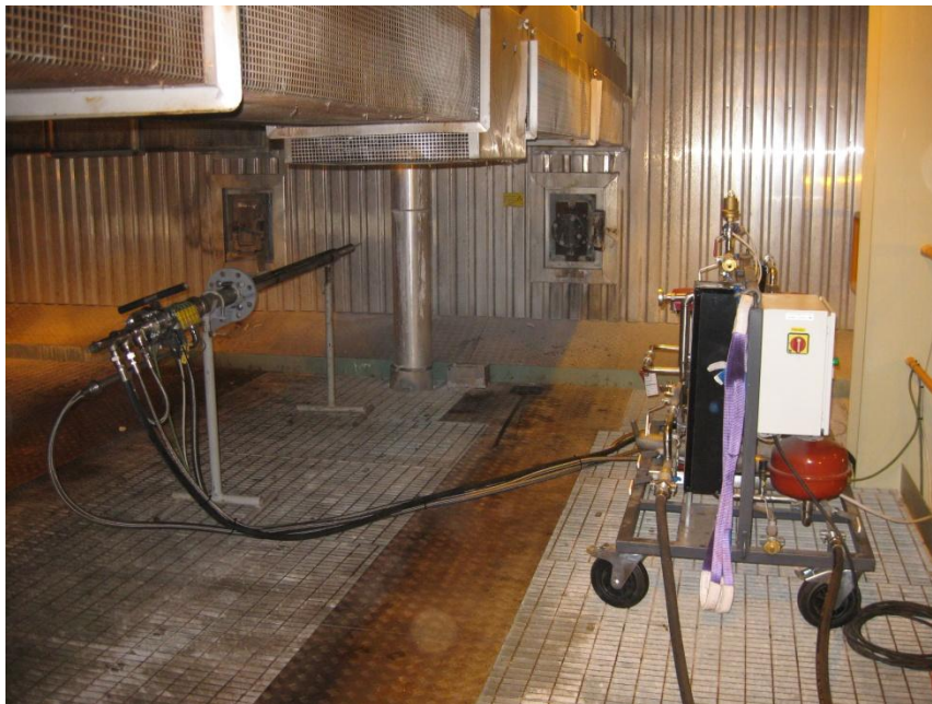
Figure 1. Probe 1 ready for insertion through an inlet located about one meter below the sootblower at level 10 ½, between 2nd and 3rd superheater.
