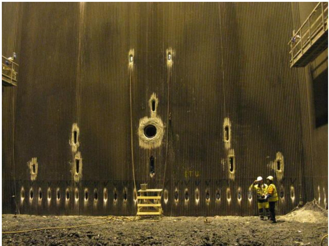
Figure 7-1. Bottom Lower part of the recovery boiler furnace with a separate incinerator for CNCG burner opening in the centre.
