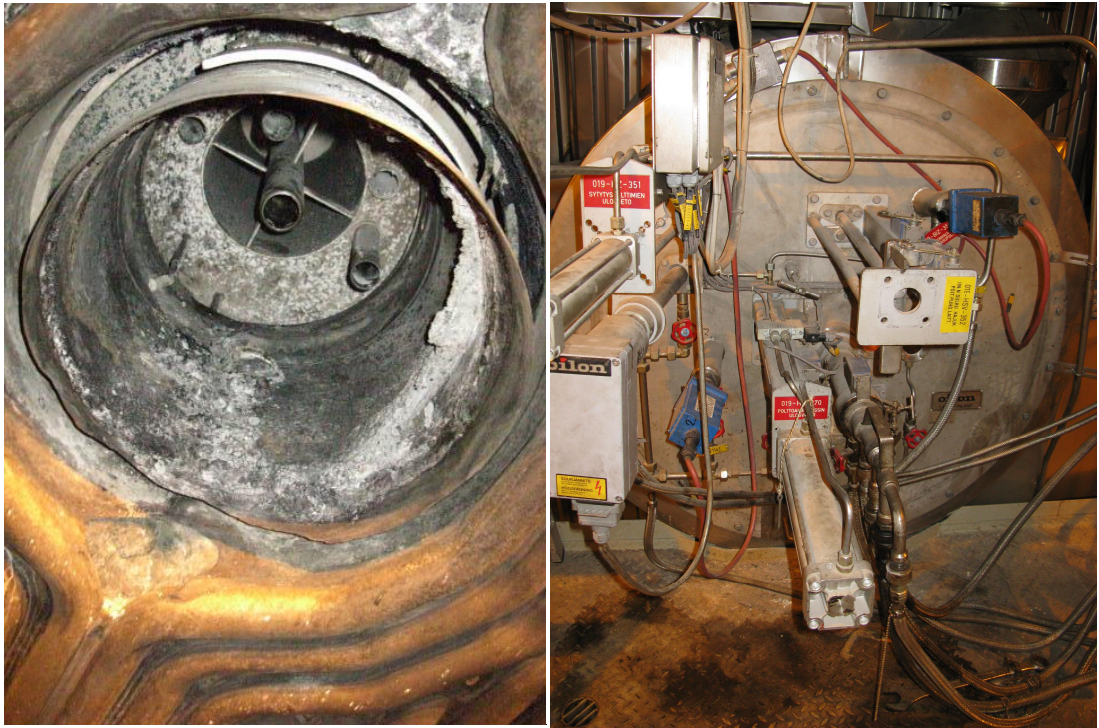
Figure 7-23. Inside and outside of a CNCG burner.
