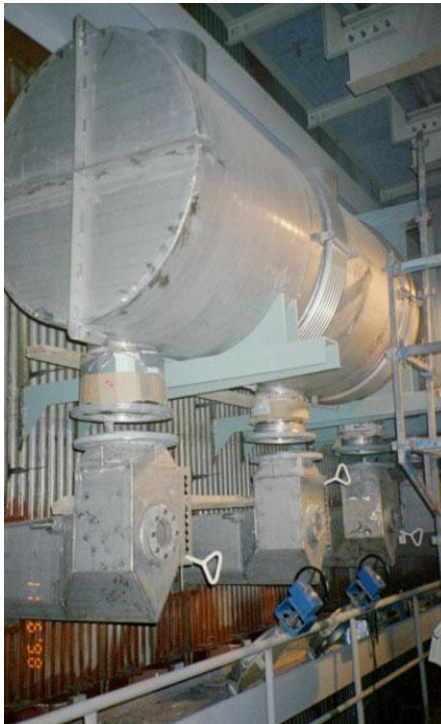
Figure 5-2. Installation of a mill's dilute non-condensable gas incineration system.
