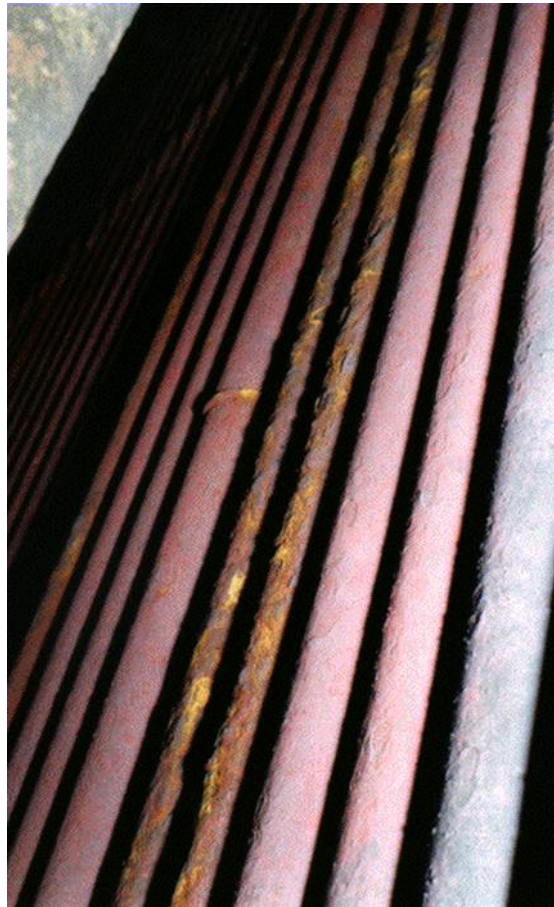
Figure 6.1. Example of chlorine induced superheater corrosion.
