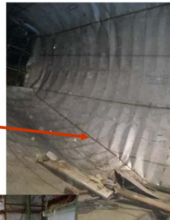
•Upper secondary air duct after explosion (inside)
