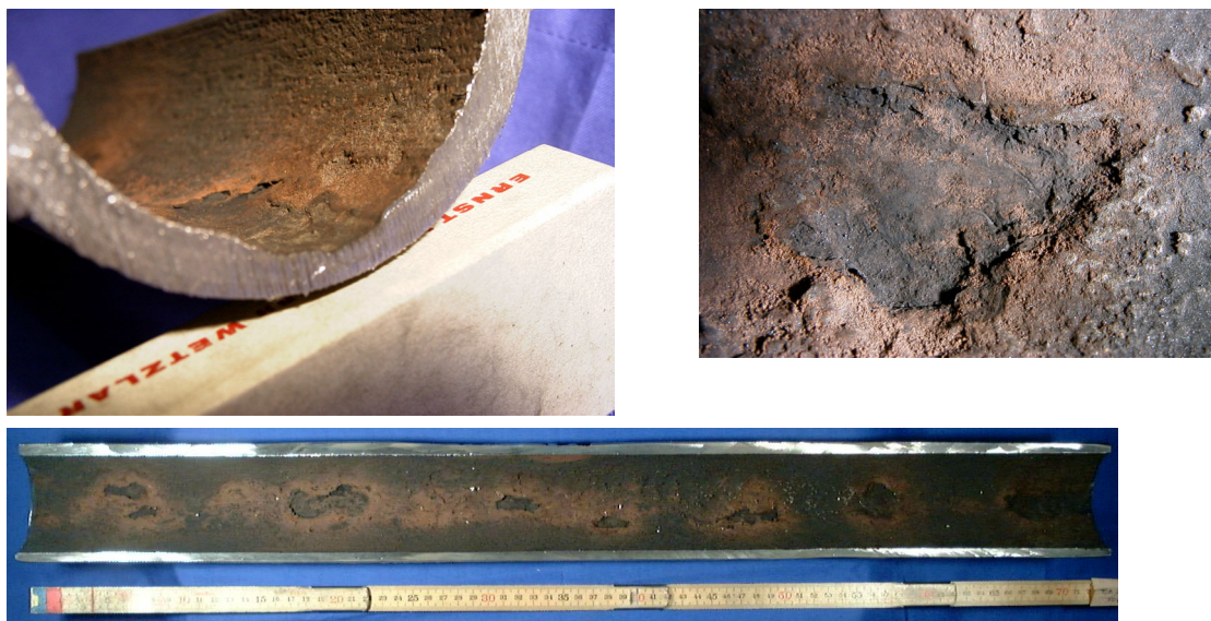
Fig 2. Pictures of the corroded tubes, Mörrum Mill.
