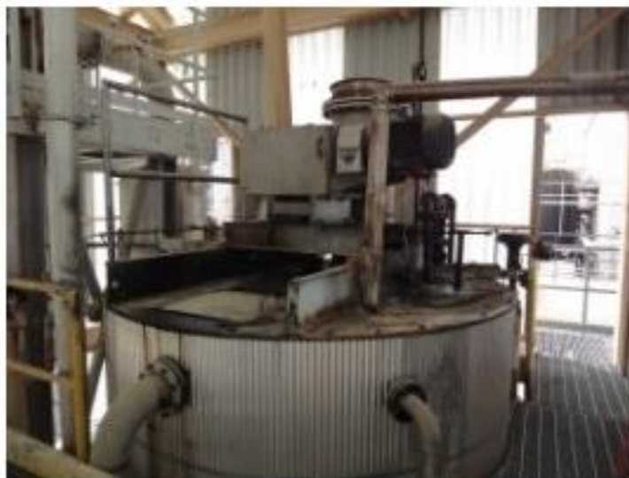
Figure 9. Photo of a soap skimmer installation [14].
