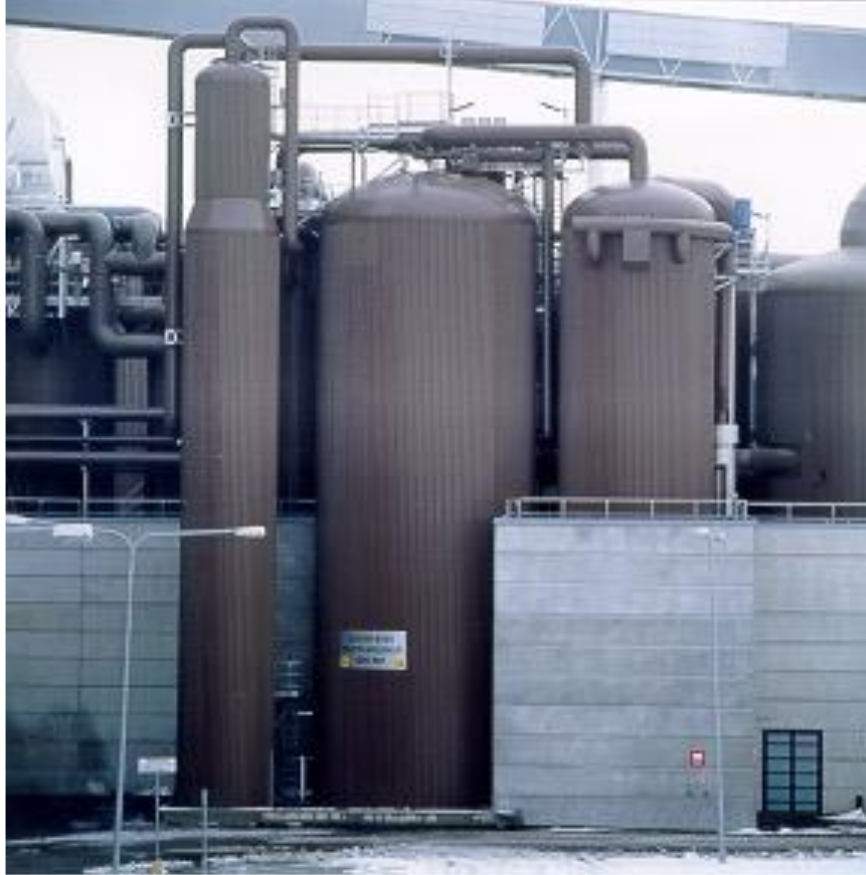
Figure 7. An industrial thermal deactivation plant for a black liquor with severe calcium scaling of black liquor evaporators.
