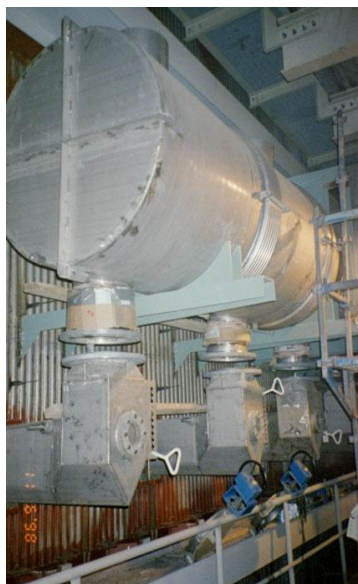
Figure 5-2. Installation phase of a mill's DNCG incineration system.
