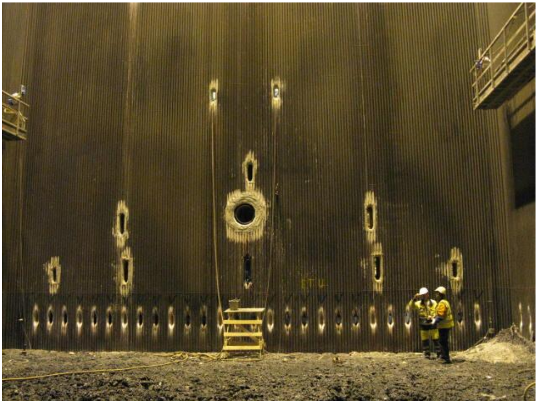
Figure 7-1. Lower part of the recovery boiler furnace with a separate CNCG burner opening in the centre.
