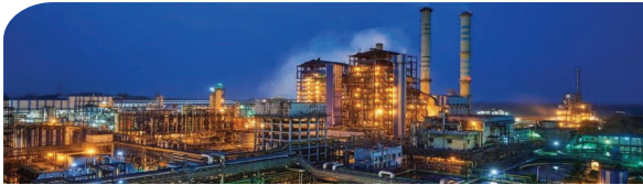
Unit Bhadrachalam, Bhadrachalam ITC Limited, India
