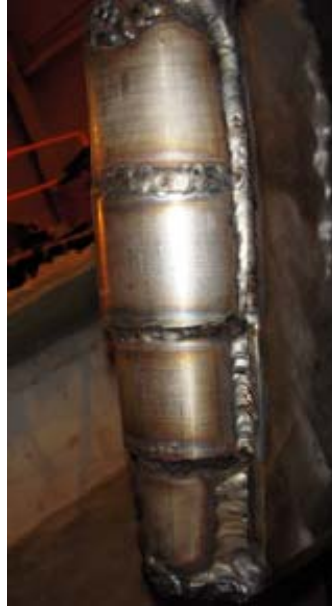
Figure 3. Steam generator front wall with tested materials
