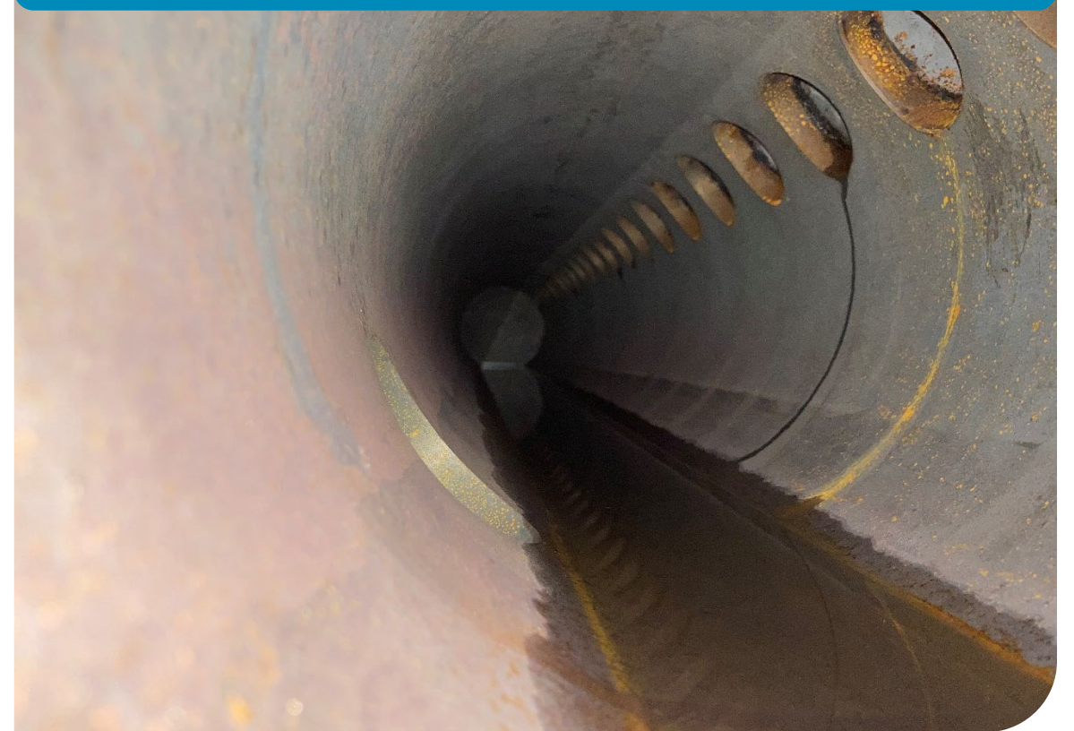
Lower waterwall header post manual flushing
