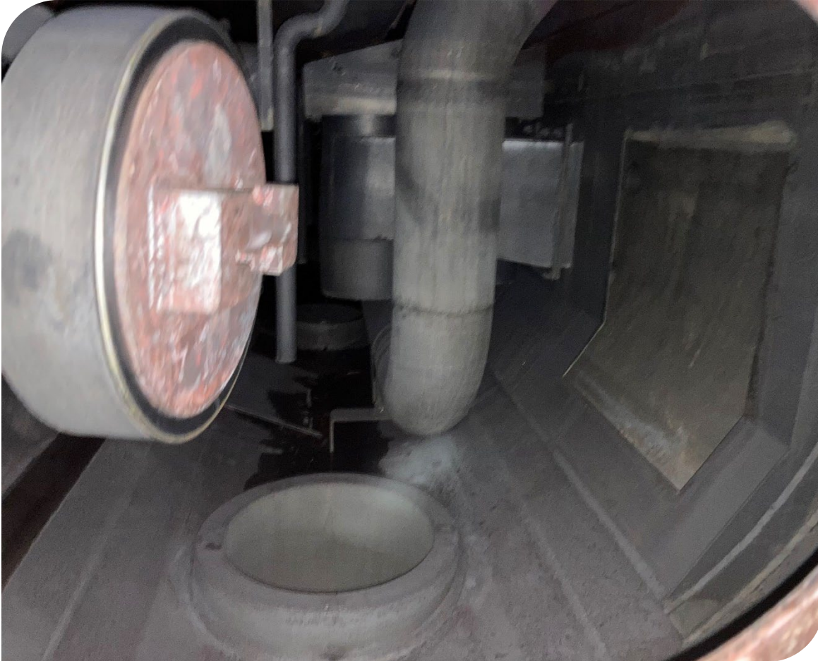
Steam drum prior to hand flushing
