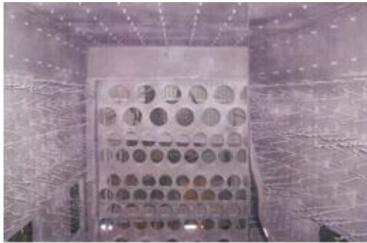
Figure 9. ITC coated steel walls behind refractory linings. (Courtesy of Viktor Anaya, FicerMex)
