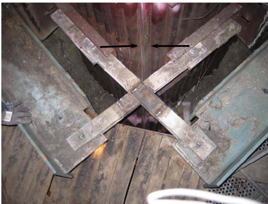
Repair by locking the bucks stays in the new position. Extended link arms and new split pins. Note the widened "double membrane" (arrows).
