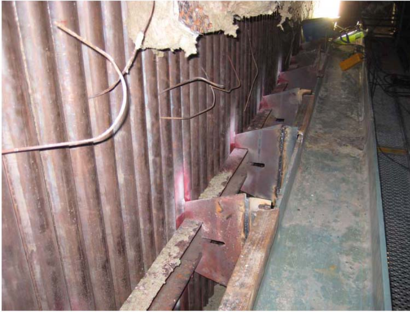
Repaired and extended connection plates, between furnace wall and buck stay.
