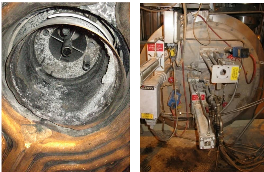
Figure 7-4. A CNCG burner photographed from inside and outside the boiler.
