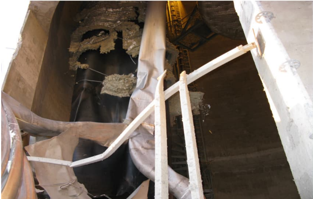
Figure 0-1. Photo of the inner stack after the explosion.
