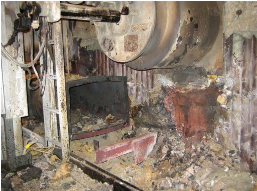
Figure 0-2. Photo of the DNCG duct after the fire.
