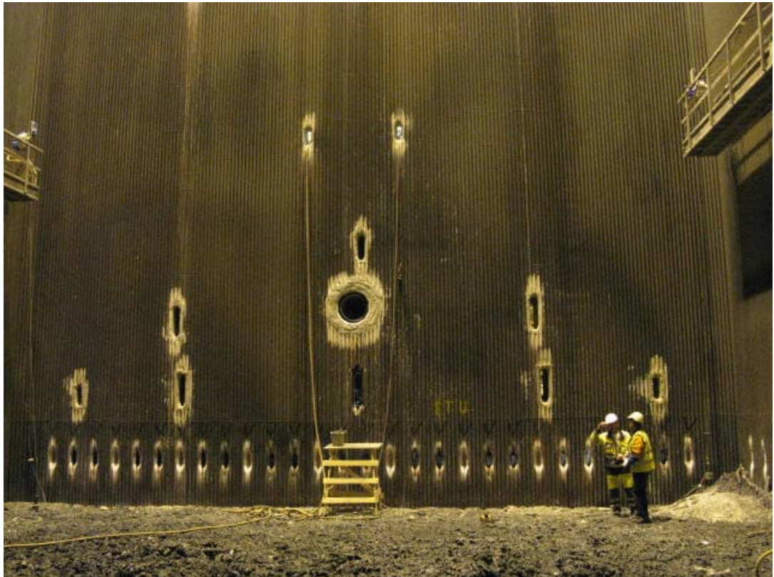
Figure 7-1. The lower part of a recovery boiler's furnace with a dedicated burner for CNCG in the middle.
